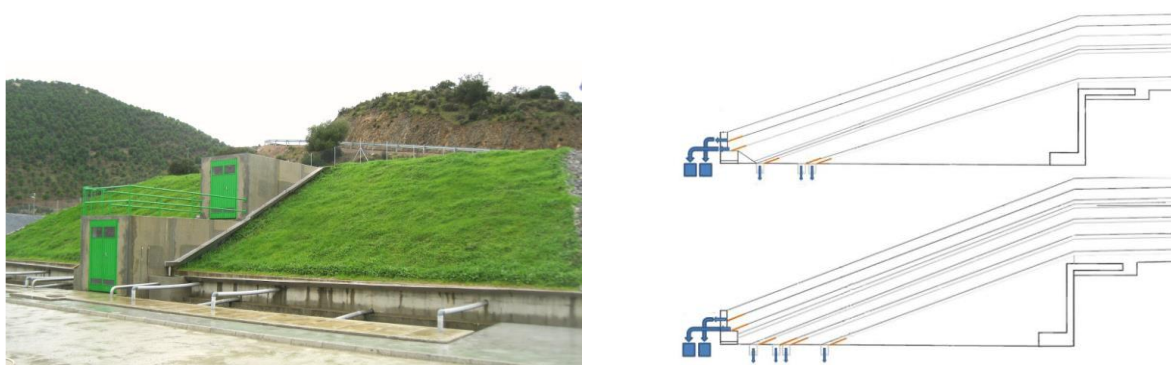
Figure 3-8 Details of the drainage water collection system of the El-Cabril mock-up cover.
