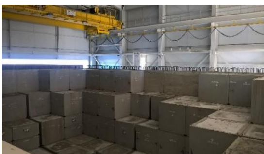
Figure 2-35 Disposal units into a vault
