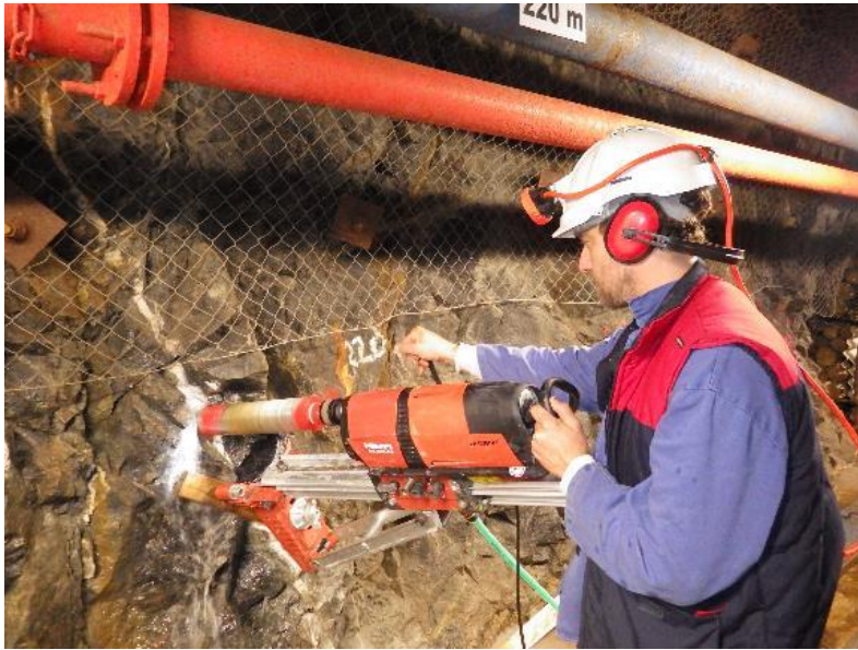
Drilling location: BZ-XIIJ_219,4 m
