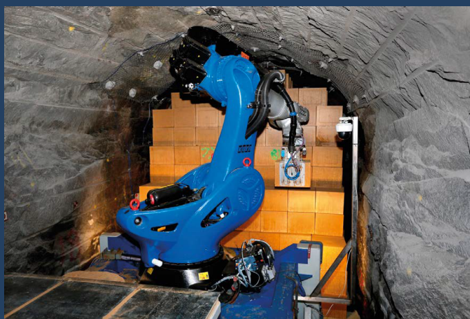
Industrial robot backfilling a gallery with bentonite blocks. Remaining voids (between the rock surface and the blocks) will be filled with bentonite pellets (source: SKB).
