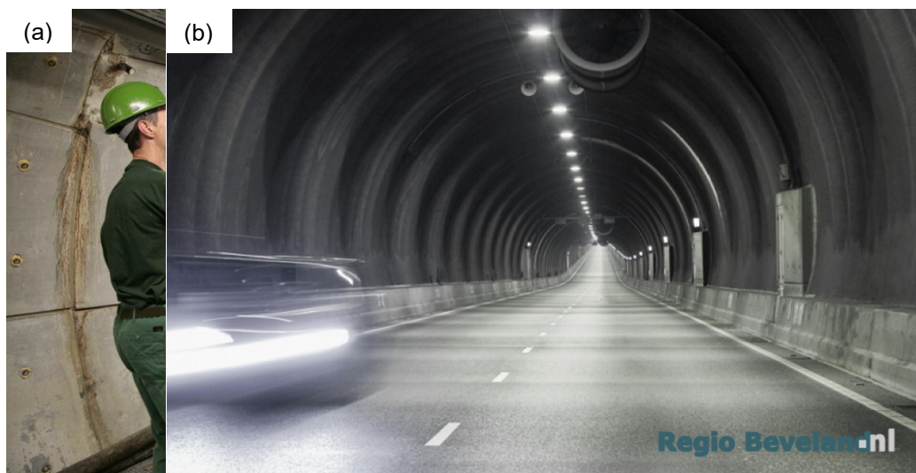
Figure 4-16 – (a) salt deposits at joints of concrete segments in HADES URL and (b) traffic tunnel – Westerschelde tunnel – constructed in Boom (Rupel) Clay in the Netherlands.
