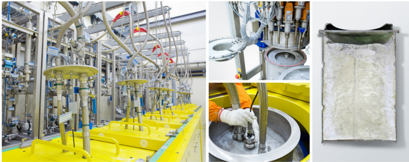
GNS drying facilities for conditioning of SIERs (source: GNS.de)
