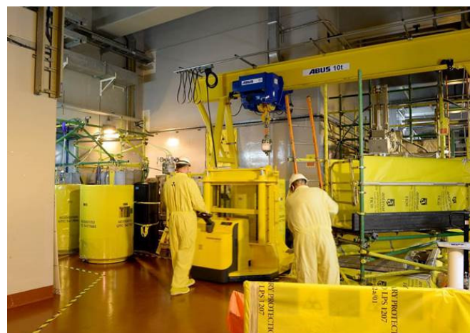
GNS NEWA & FAFNIR facilities in operation for drying of MOSAIK® II drums (source: gns.de)
