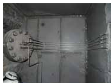
Pressurization pipes mounted onto the concrete backwall surface and passing through a flange of the rock lead-through pipes
