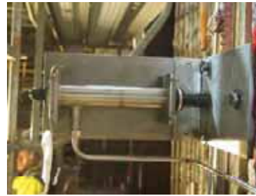
Displacement sensors at the back face of the plug and specially designed sensor holder
