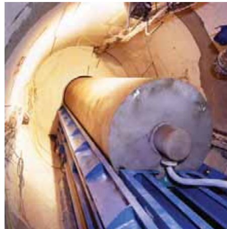
Disposal in horizontal drifts
