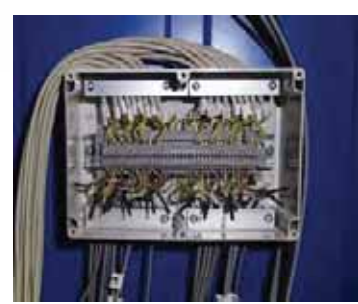
Leakage box for interrupting potential water leakage along and inside the wires
