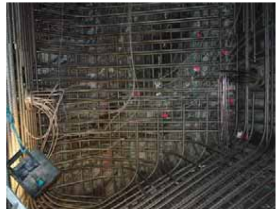
PVDF and stainless steel tubes, directing the pressure sensor cables to the cable flanges towards the filter layer (right side) and plug section 2 (left side)
