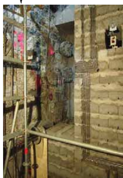
stainless steel tubes for hosting the sensor wires, mounted onto the filter layer wall
