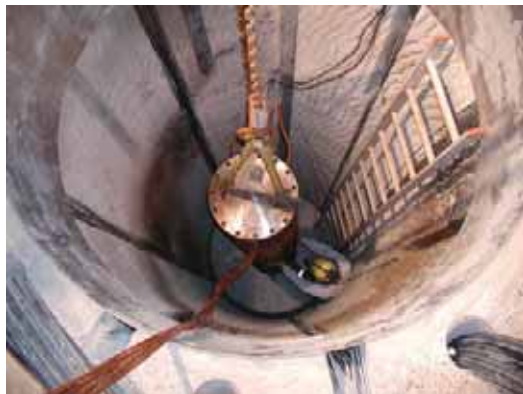
Disposal in vertical boreholes
