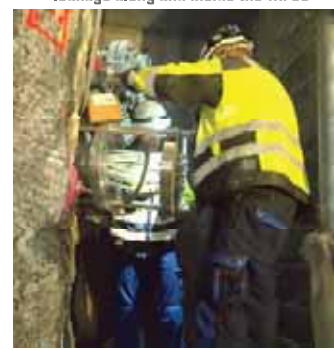
Leakage box for interrupting potential water leakage along and inside the wires
