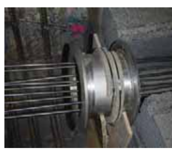
Wire flange for sealing of cables passing between filter layer and plug section 1 during construction
